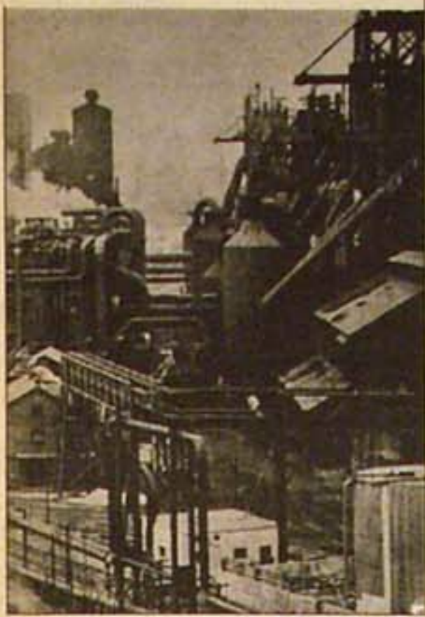
Cleveland steel plant.
